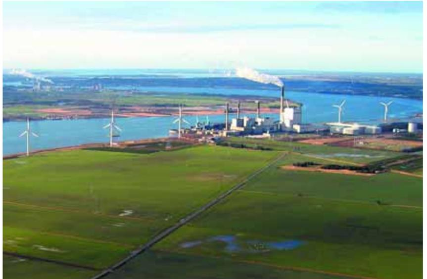
Technologies continue to be developed to improve the environmental performance of coal fired power stations – the Nordjyllandsværket coal fired power station in Denmark has an efficiency level of 47%. Photograph courtesy of Elsam. Photographer Gert Jensen.
