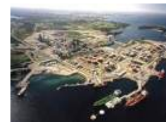
Statoil Mongstad Norway - 40 MWth Chilled Ammonia - Gas
